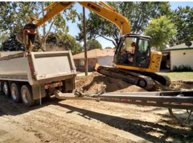
Phase 2 - cut out excess soil and haul it away.
