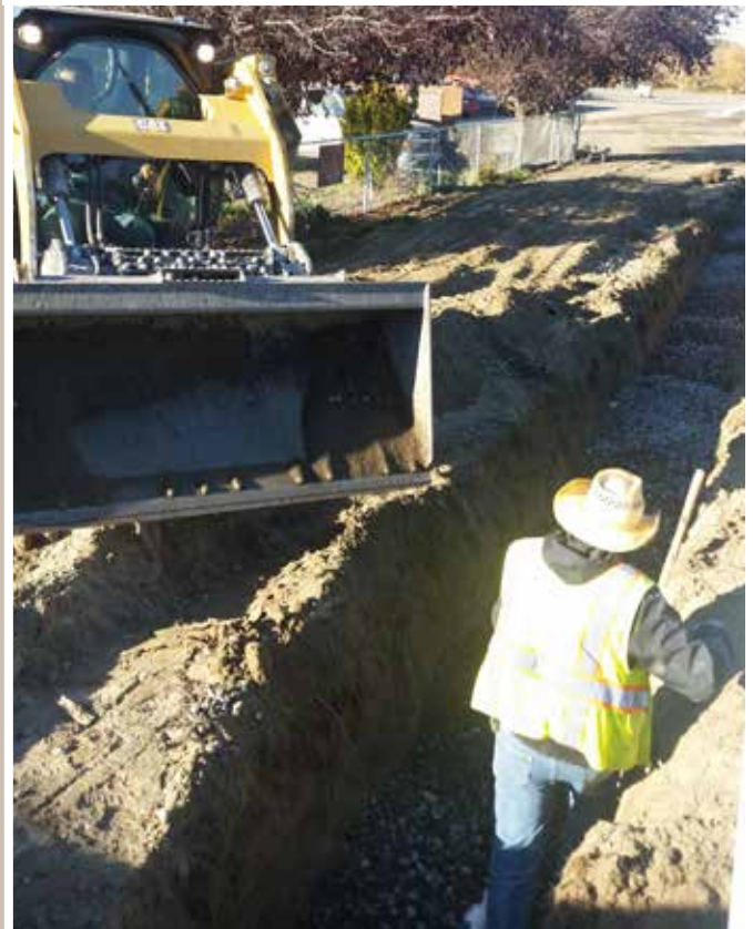
Nate is putting the final touches on this drain field prior to installing the rock. Below: Sal operates the skid steer in tight quarters under Nate's watchful eye!
