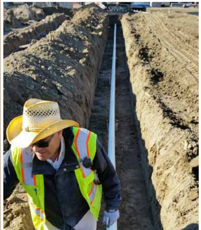
Nate is putting the final touches on this drain field prior to installing the rock. Below: Sal operates the skid steer in tight quarters under Nate's watchful eye!
